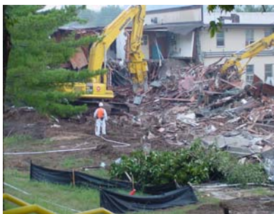
Demolition of ORNL Bldg. 1000
