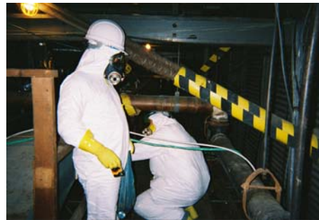
GEM Structural Engineer and ES&H Officer Assessing Hazardous Materials & Structures
