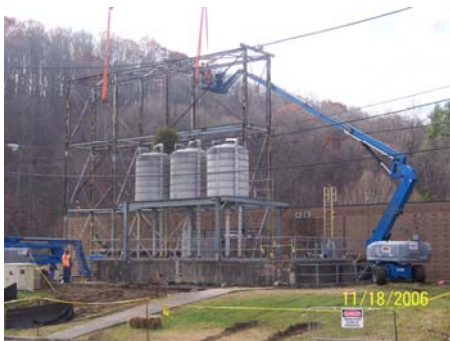
Experimental Structure Demolition
