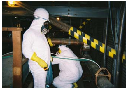
GEM Personnel Assessing Hazardous Materials & Structures
