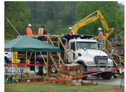
Crews Burrito Wrap Non-Friable Asbestos Waste
