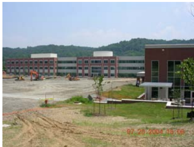
ORNL Main Entrance Under Construction
