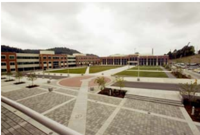
ORNL Main Entrance Construction Completed
