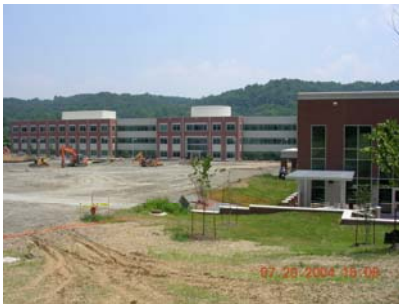
ORNL Main Entrance Under Construction
