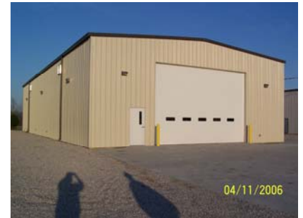
BGAD Container Repair Facility
