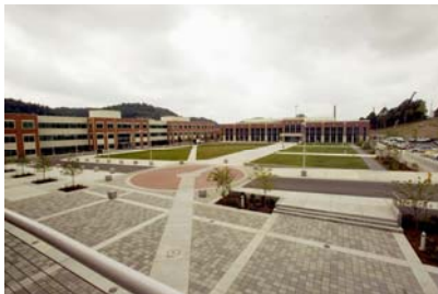
ORNL Main Entrance Construction Completed
